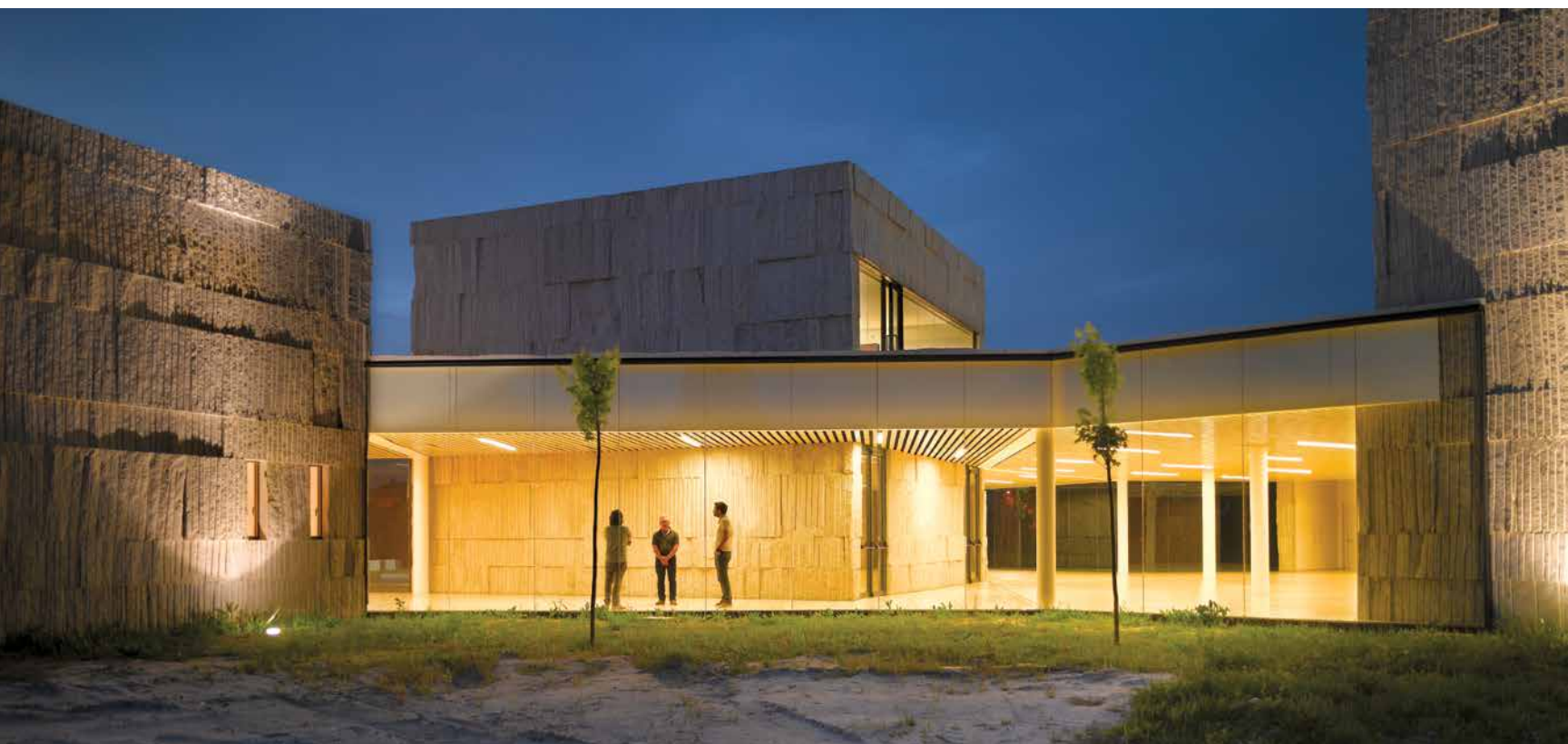
VERIN ARTS CENTER The project offers the intimacy of a house and the heterogeneity of a small town. The displacement and delicate turns of a series of volumes—which house a lobby, galleries, a large theater, and a restaurant—produces a seemingly random plan and appearance, but highly flexible spaces of varying scales.
