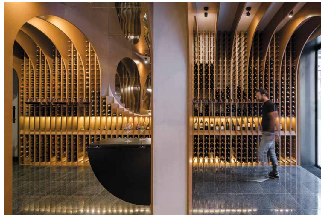
DE VINOS Y VIANDAS The architects used three materials for this winery: wood for the ribs that reference wine barrels, stone for the floor like that in antique cellars, and a mirrorlike material that creates reflections throughout the space.
