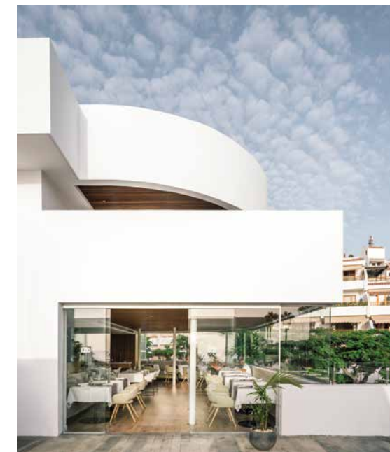
FLAMINGO CLUB In this renovation, the structure is set back from the facade, where curving horizontal bands create a smooth transition between the contrasting, more orthogonal north and south elevations over a steep slope.
