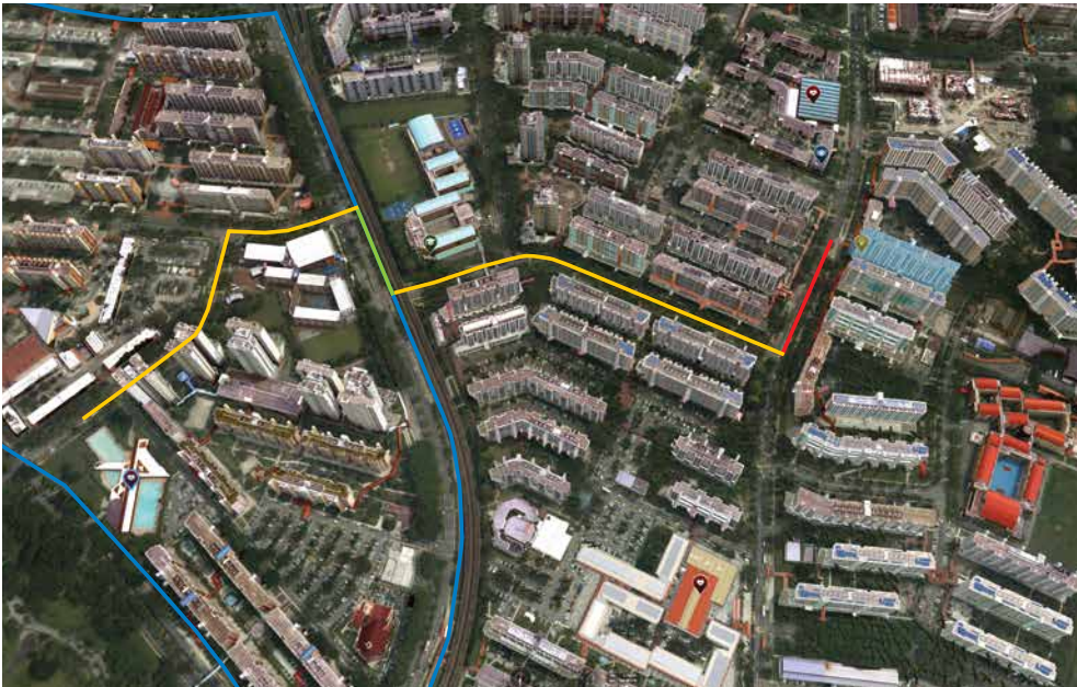
Virtual Singapore, a synthesis of the digital models of various government agencies and vast stores of data, can be put to a wide variety of uses, including producing a visual display of apartment resale values (top), or helping bicycle commuters map the best route between two points (bottom).
