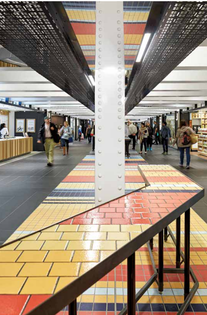
Colored tile indicates areas where pedestrians and shoppers can pause, eat, and chat (above). Overhead, a spine of mirror and perforated metal screens—laser-cut to reference historic subway-tile motifs—conceal m/e/p components. Backlit storefront signage (top, right) keeps the design cohesive. Small kiosks at the center are rented by niche vendors.
