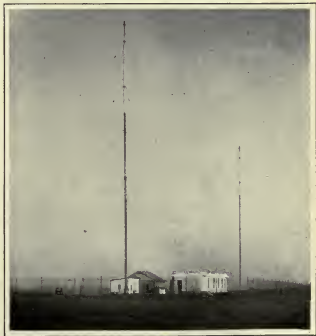
ANTENNA SYSTEM OF THE PRAGUE RADIO STATION This broadcasting station is a standard Western Electric 5 kw. outfit. The antenna is described as an Alexanderson type with three leads
