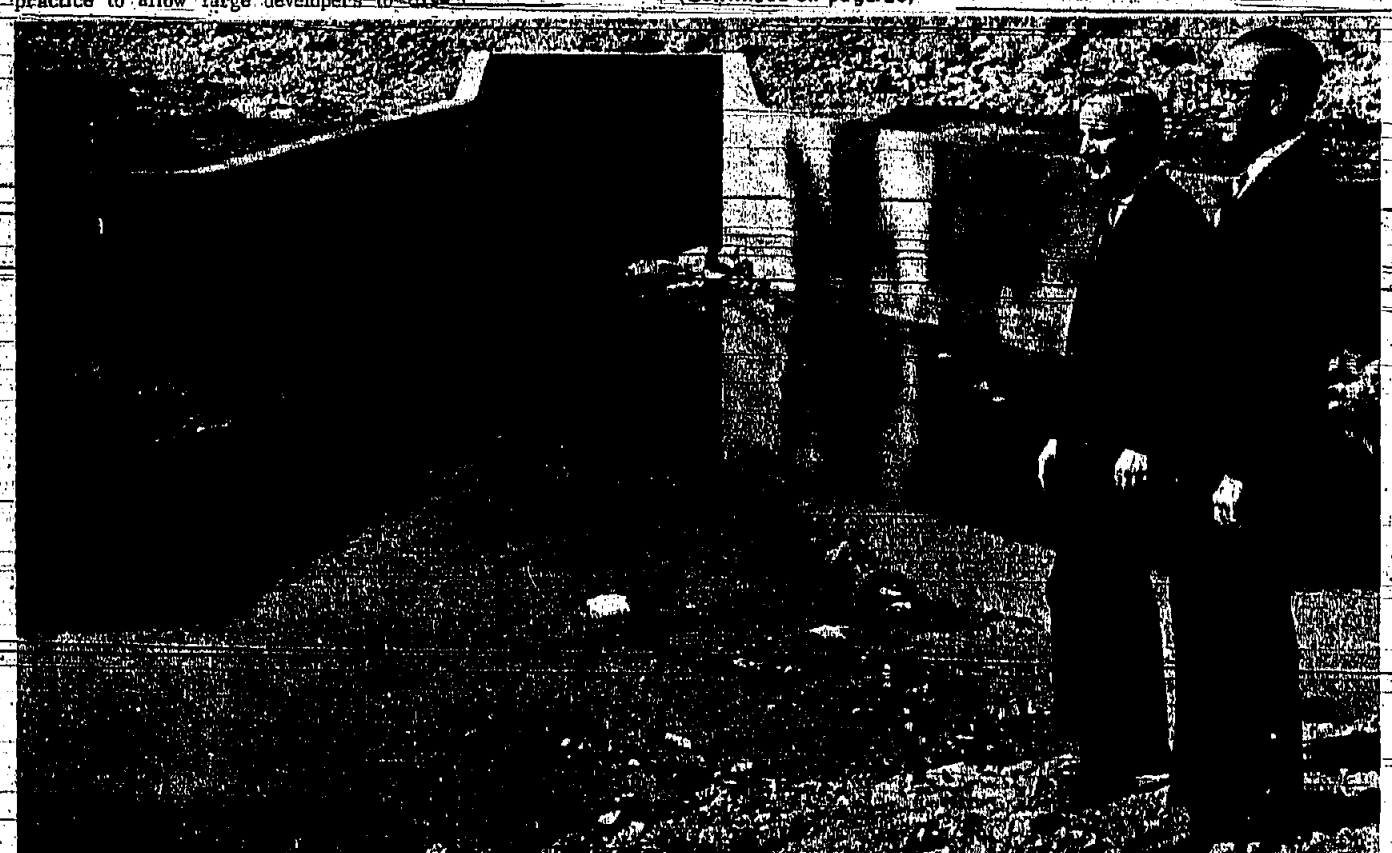
ON-SITE INSPECTION - Mayor Philip Del Vecchio, left, Republican candidate for reelection to the Township Committee, joins Congressman Henry J. Bulman in examining one of the culverts which have led to local flood problems.
