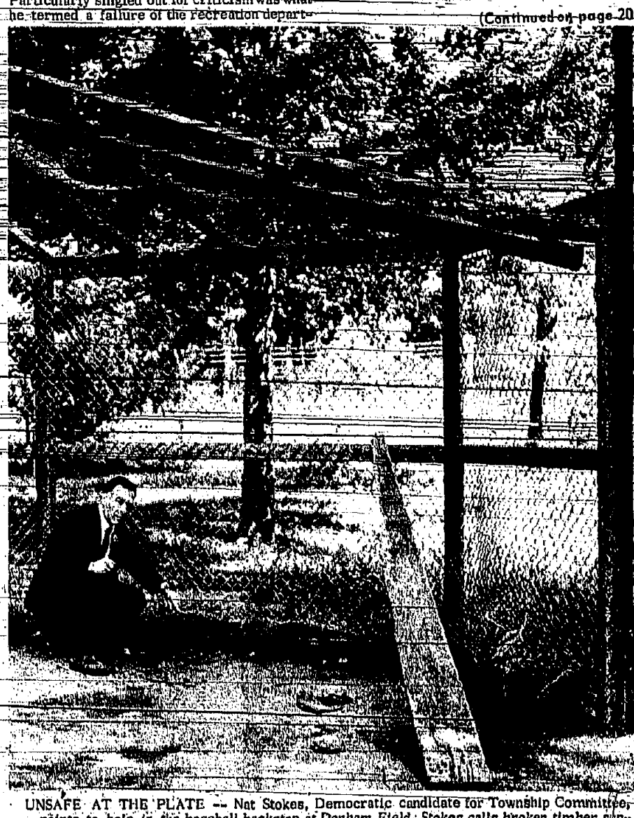
UNSAFE AT THE PLATE - Nat Stokes, Democratic candidate for Township Committee, points to hole in the baseball backstop at DeWitt Field. Stokes calls broken timber supports and protruding wire ends a hazard to players, calling for constant maintenance of athletic facilities.
